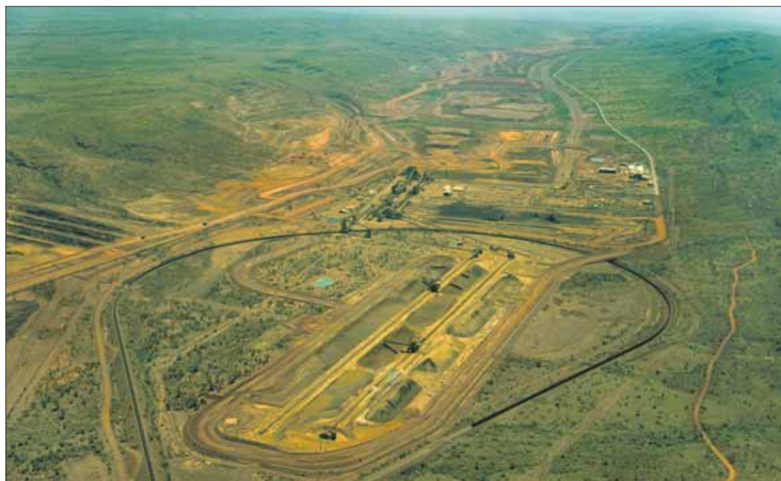
Powerhouse: BHP is going to build and operate a CCGT power station in Newman to power its Pilbara mining operations.
